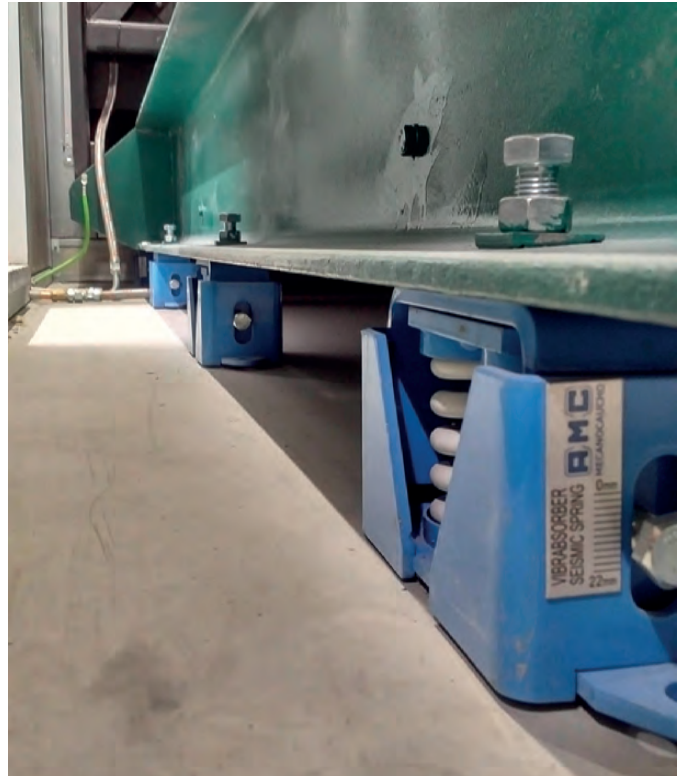
Compressor insulated with VIBRABSORBER +Sylomer®
