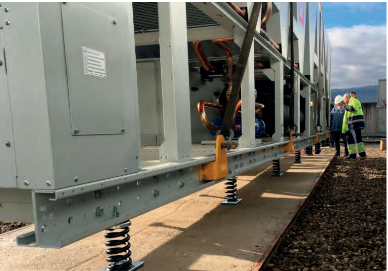
Ventilation system insulated with VIBRABSORBER
