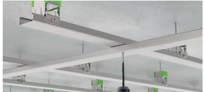
10.- Place transverse profiles in position.
