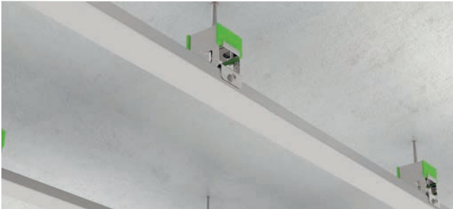
9.- Acoustic hangers and profiles fixed.
