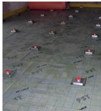
Conditioning the premise and installation of the mounts.
