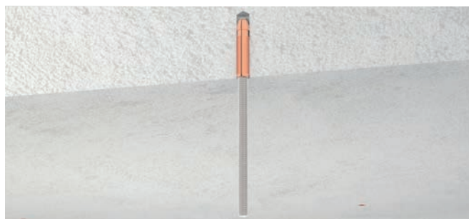
4.- Level the hangers using a laser alignment tool.
