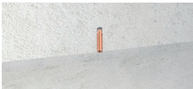
3.- Attach the acoustic hangers to the end of the studbolt.
