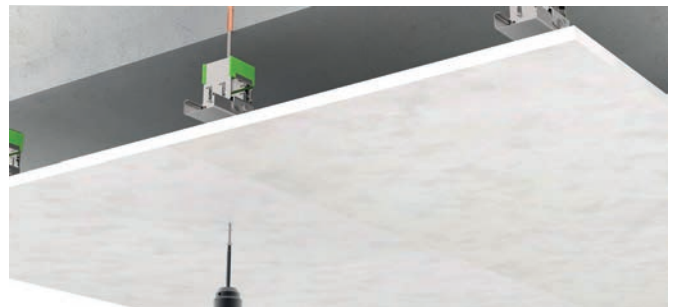
12.- Position plasterboards in place.
