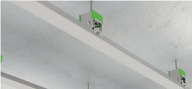
9.- Acoustic hangers and profiles fixed.
