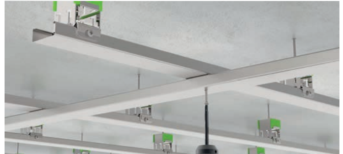
10.- Place transverse profiles in position.
