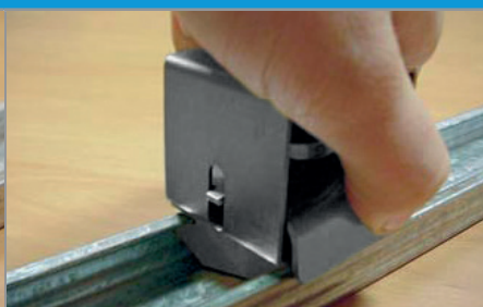
2. Turn the part inside the beam until it is fixed.
